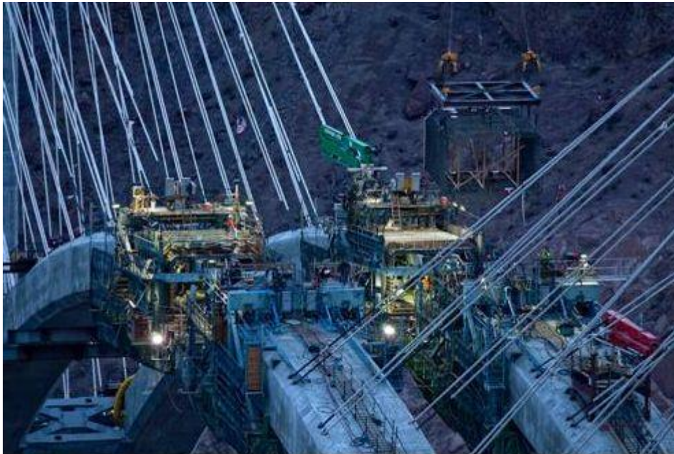
Joining requires extremely careful work! (c) Jamey Stillings Photography
